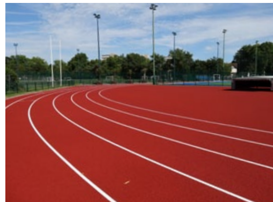
Resurfaced porous macadam track
