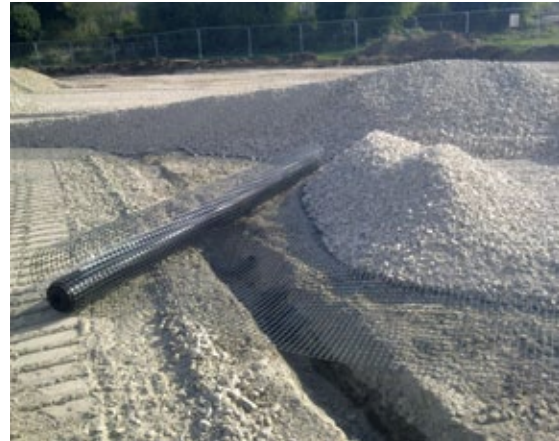
Plastic mesh within stone layer
