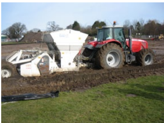
Installation of ground stabilisation treatment
