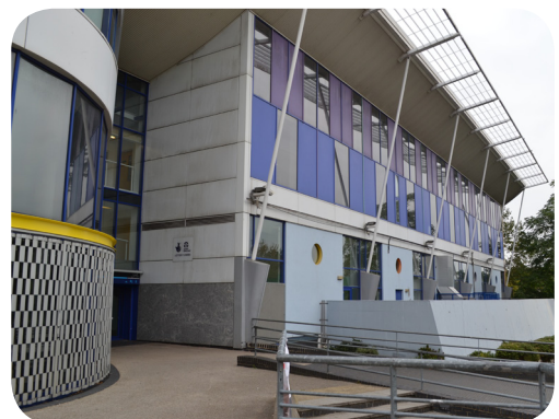
75 m 2 of solar panels to be installed on the roof
