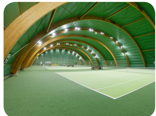
New playing surface and LED lighting to indoor courts
