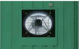
High-level radiant heaters on walls and extract fans at ends of the building
