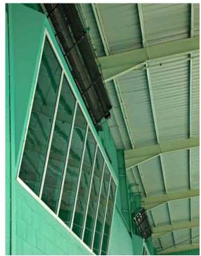
Informal spectator gallery screened using tinted glazing at an angle to minimise distraction and reflection
