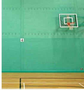
Acoustic blocks used in the wall construction
