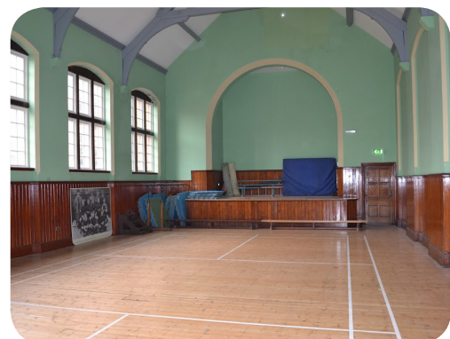
New heating for concert hall with recessed radiators
